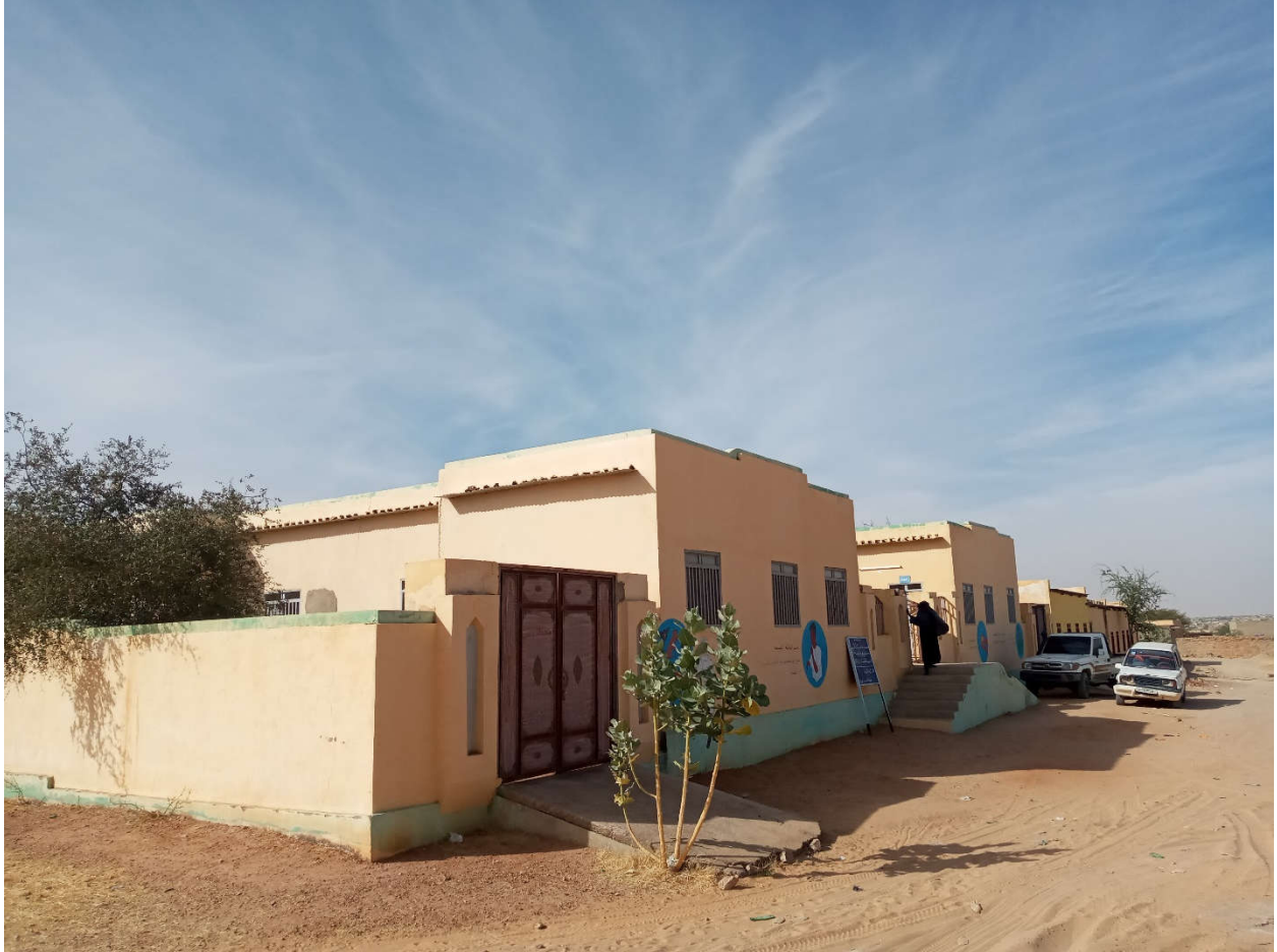
Figure 1. Hospital View from the Northern Side
